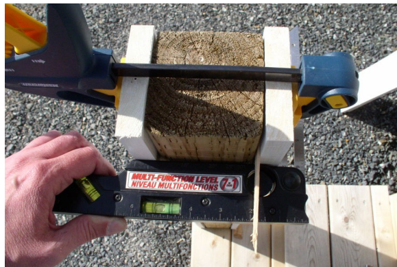
Fig. 5 Use shims to keep boards straight and square to each other.
