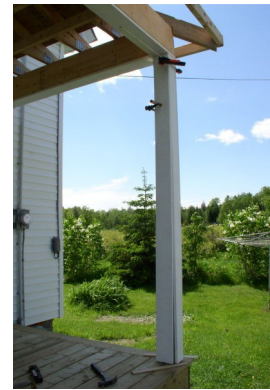
Fig. 6 The bottom of this board was out of alignment so I used clamps & blocks to force it into position for nailing.
