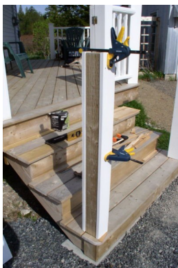
Fig.4 Clamp face boards to the post
